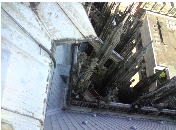
Illustration 14: cable drop from the intersection spire, with rubber edge protection.
